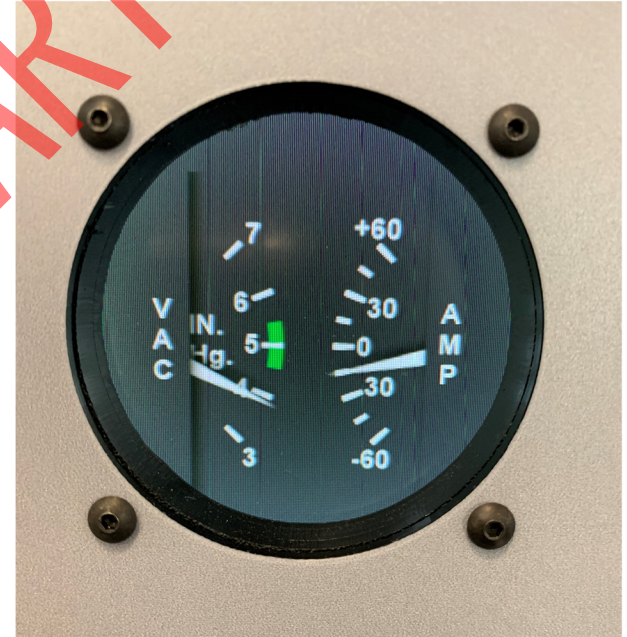
Ammeter showing a discharge
