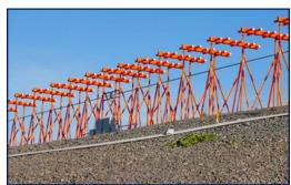
Figure 15: Localizer Antenna (LOC)
