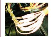
Unsupported wiring with excessive tension at connections
